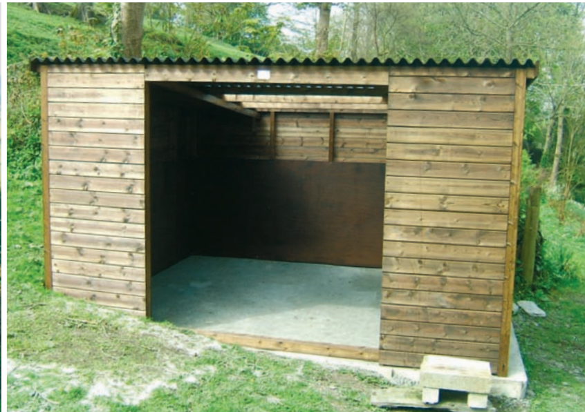
10' x 12' pony shelter with the boarding on the outside, kicking boards inside and 2 clear roof sheets
