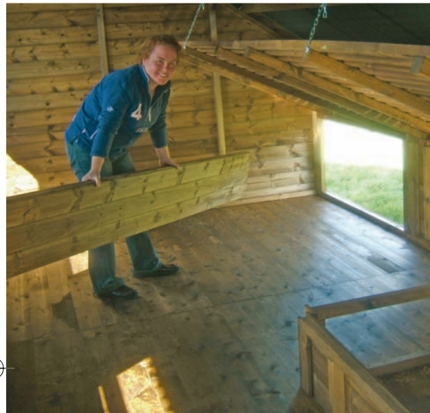
Removable perch benches for easy cleaning
