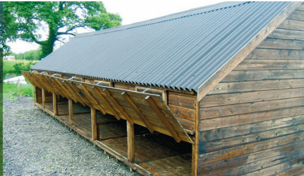
Needwood 300 bird house showing rear cleaning shutters
